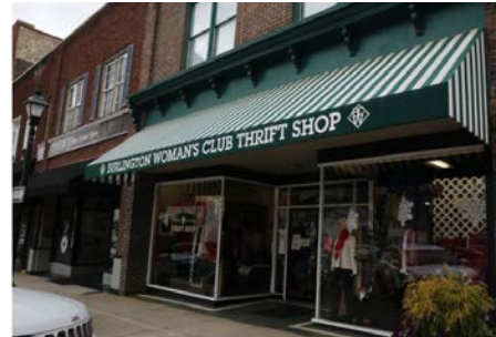
Awning with signage along valance
